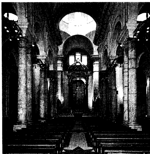
Figure 9 Basilica di Bonaria: church interior showing the twin columns in limestone blocks and the overhanging reinforced concrete slabs, Cagliari, 1990
