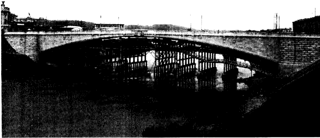
Figure 4a View of the Risorgimento Bridge, before striking the reinforced concrete centres, Rome, 1911. (APT)
