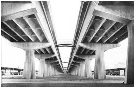
Figure 6 The Corso Francia Viaduct, Rome 1958–60 (Nervi 1963)
