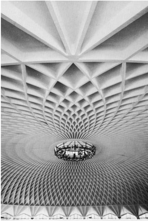
Figure 2 Small Sports Palace. The dome from the interior (Nervi 1963)
