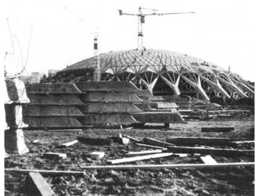
Figure 7 Small Sports Palace: view during construction of the dome (Nervi 1965a)
