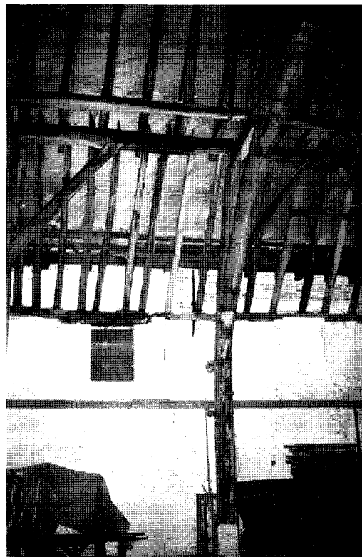
Figure 9 Saint John's hospital Bruges, roof construction of the middle hall, 1234 \pm 6 (d). (Photo by the author 1999)
