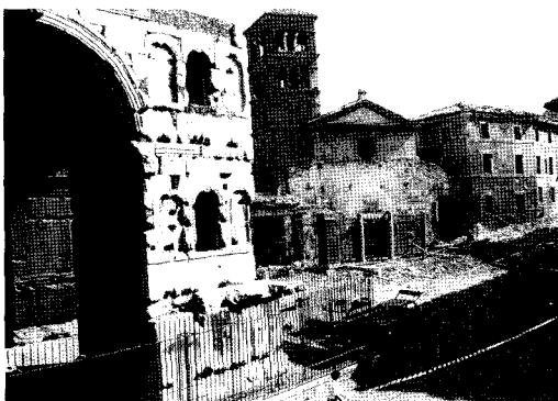
Figure 7 The complex building articulation has appeared in the front of the church, under the fallen plaster following the explosion caused by the terrorist attack (Author's photo)
