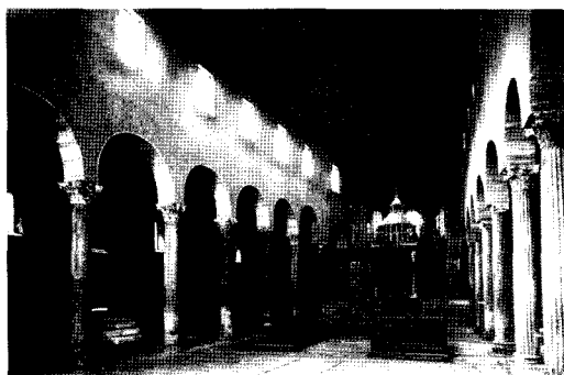
Figure 6 The church, inside, after the intervention of Antonio Muñoz (1924–1925) (Muñoz 1926, pl. XXXII)
