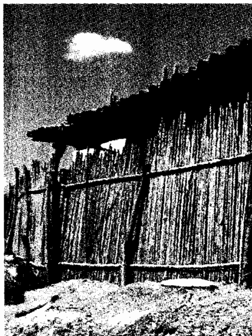
Figure 2 Primitive South America: Traditional hut showing bahareque or quincha wall construction (from Federico Vegas, Venezuelan Vernacular , 1985)
