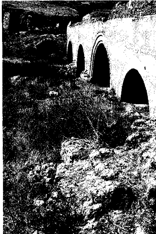
Figure 4 Bridge of Carmona
