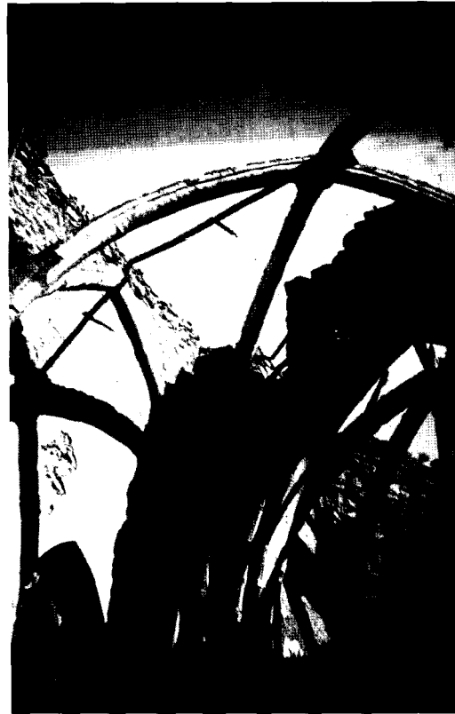
Figure 4 Ribs of a vault after the collapse of the compartments (document : Anne Coste)
