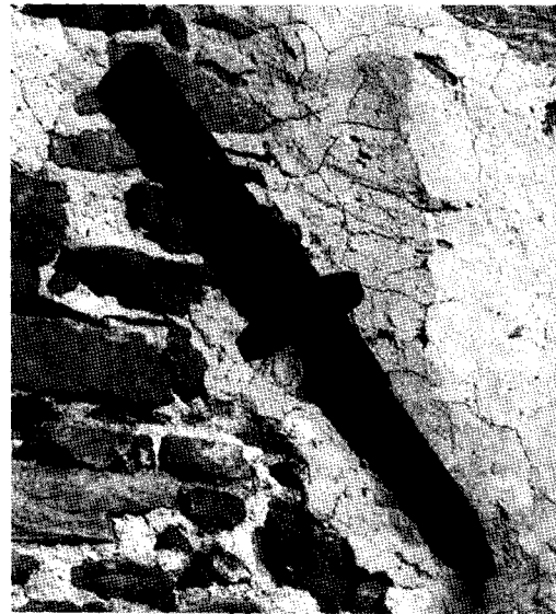
Figure 3 Tie beam anchorage (type n.2)
