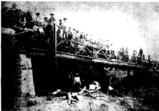
Figure 6 Unidentified Runyon bridge with «crossing fan» cable pattern (HAER TX-36, photo 14)
