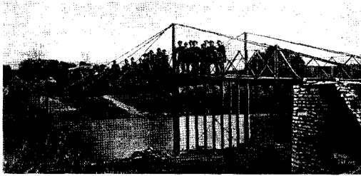
Figure 10 Whitewater River bridge by J. Mitchell at Richmond, Indiana (Bridges over . . . 1899)
